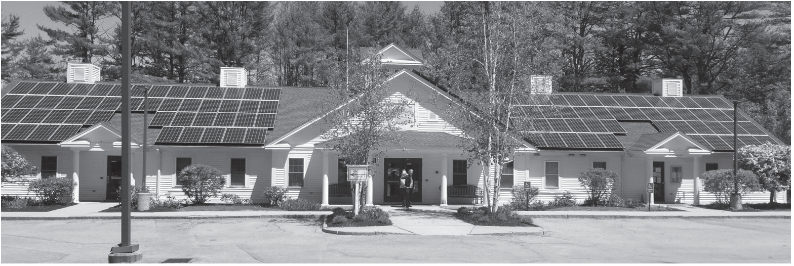
A new 33 KW solar PV array is the centerpiece of energy efficiency improvements at the Whole Village Family Resource Center.
