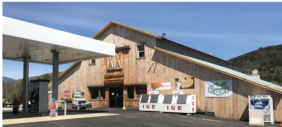
The south-facing roof of Appleknockers General Store in Warren will host the next community solar array to be built by NH Solar Shares.
