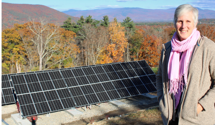
Sandra Jones and NH Solar Shares are preparing to cut the ribbon on their third community solar array, this one in Center Harbor.
