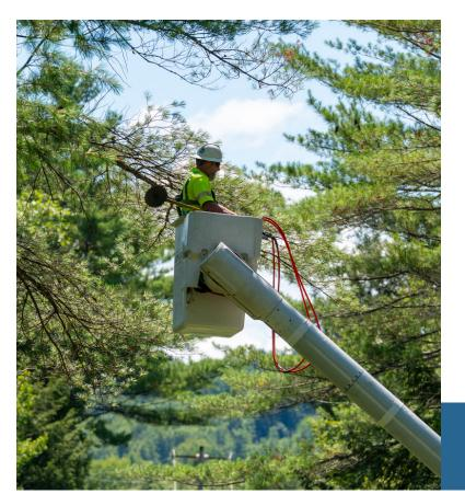
Keeping powerlines and rights-of-way clear begins with mechanical cutting of branches and trees. A year or two afterwards, when there is resprouting from hardwoods, a controlled, selective low volume herbicide is applied directly to the so-called incompatibles. The surrounding low growing species are not sprayed, allowing them to flourish and spread so that compatible vegetation naturally manages the area by outcompeting the incompatible species.
